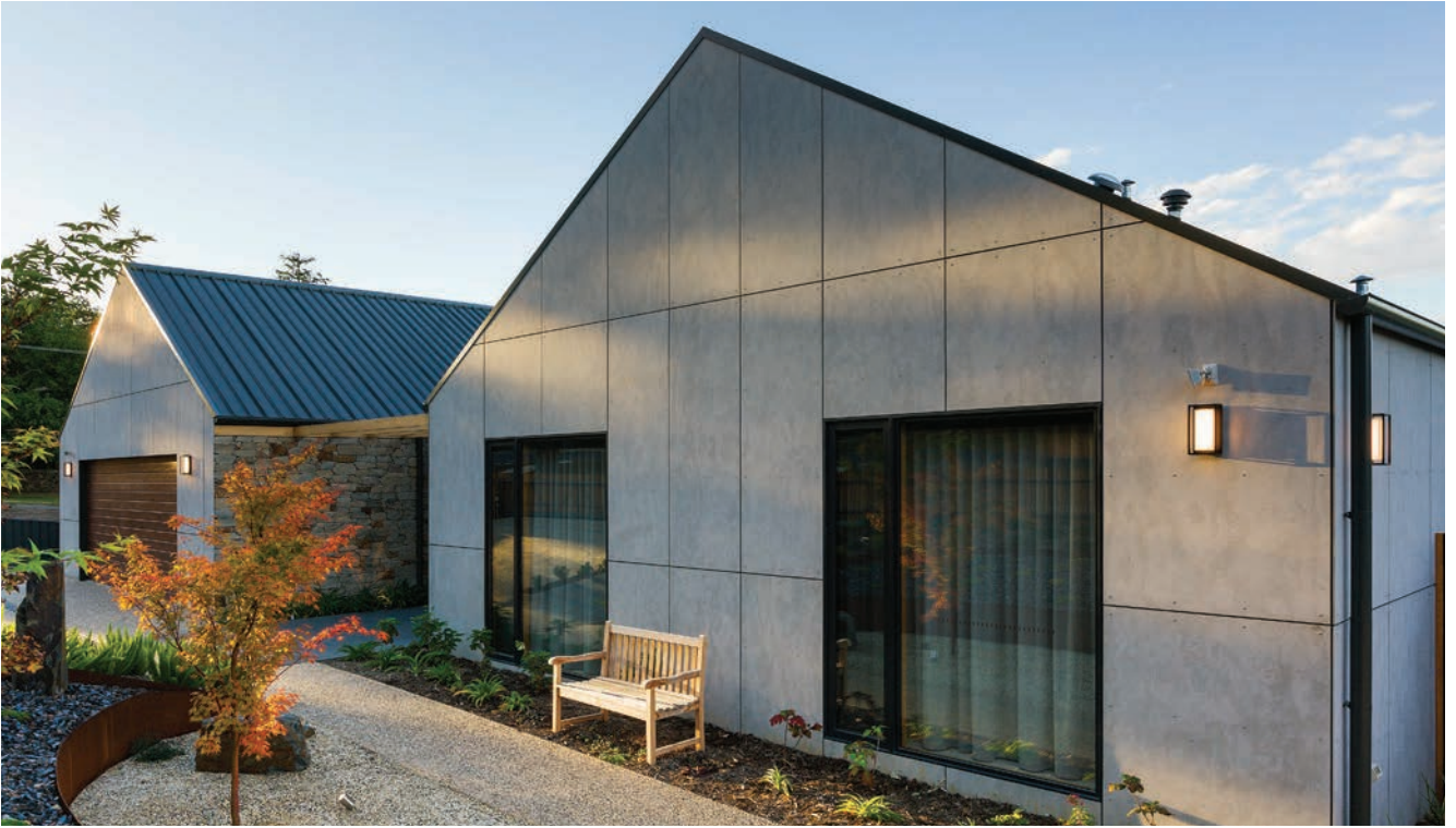
FIGURE 2.01 Barestone External and Surround on Timber Battens Overview
