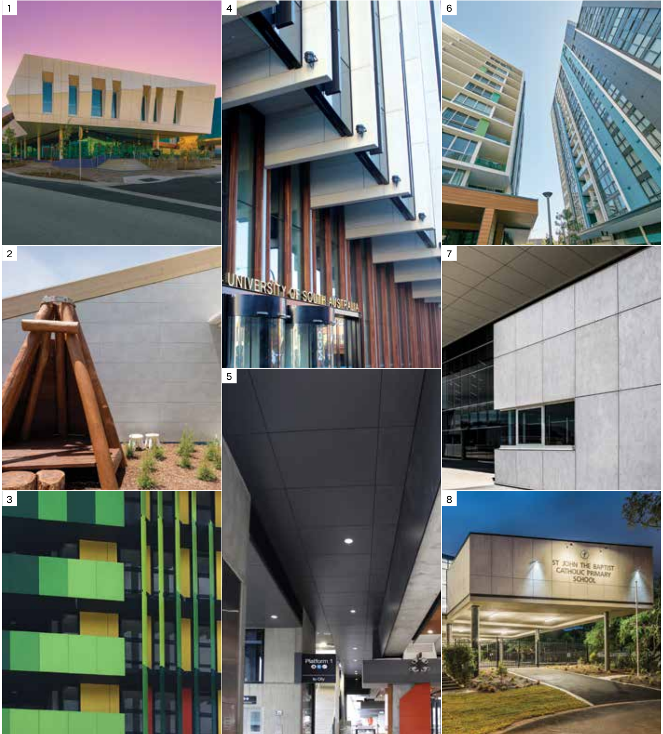
1 Casey Hospital, VIC 2 Maragon Early Learning Centre Wellard, WA 3 Commonwealth Games Village, QLD 4 University of South Australia, SA 5 Rosanna Train Station, VIC 6 Wollie Creek Apartments, NSW 7 Emmanuel College, VIC 8 St John The Baptist Catholic Primary School, NSW
