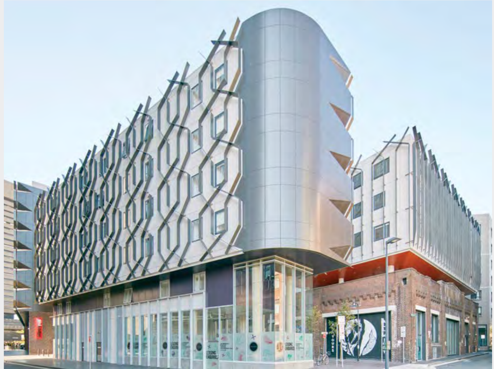
Architects: Tonkin Zulaikha Greer and Paul Davies Architect.
